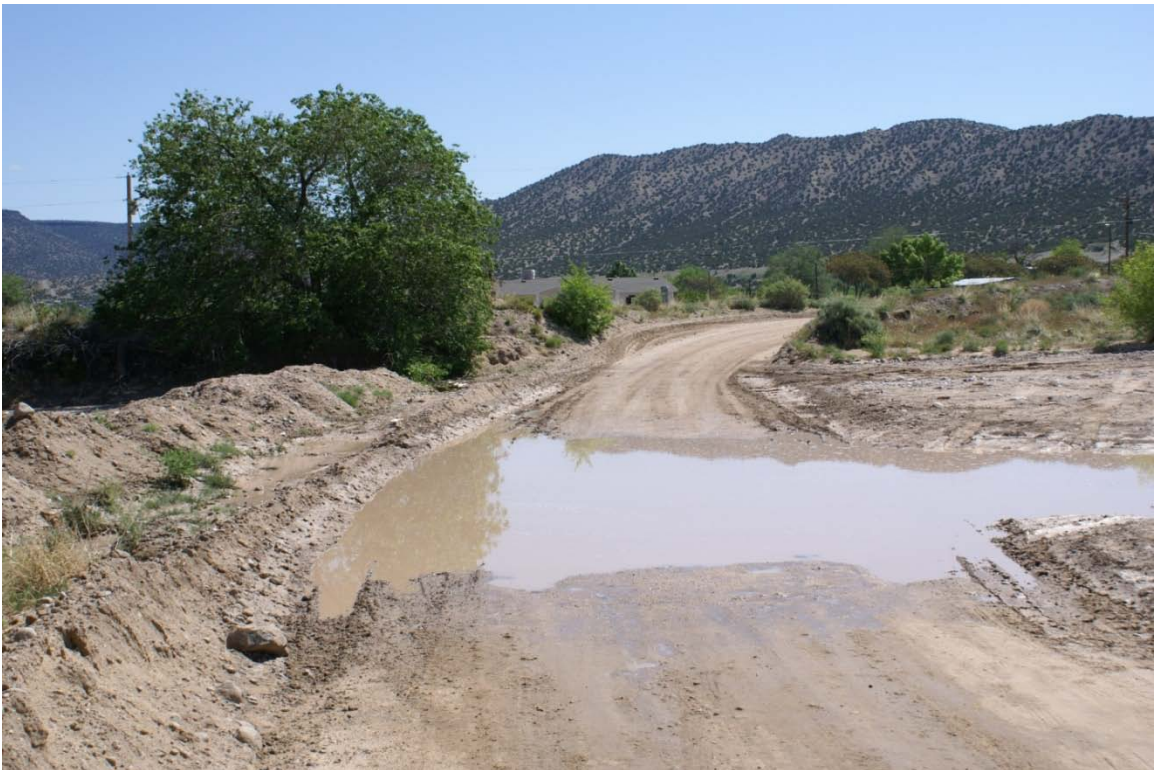
Figure 5 Flooded arroyo in Alcalde. (Johnston, 2007)
