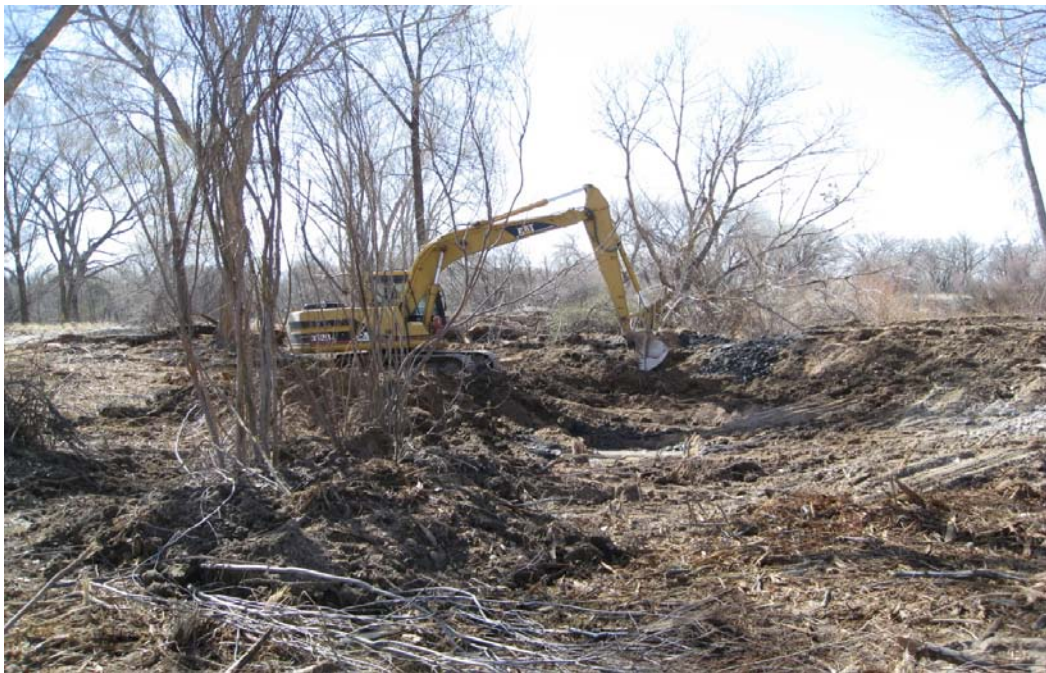
Figure 38 Maestas Property, wetland swale excavation. (McGraw, 2008)
