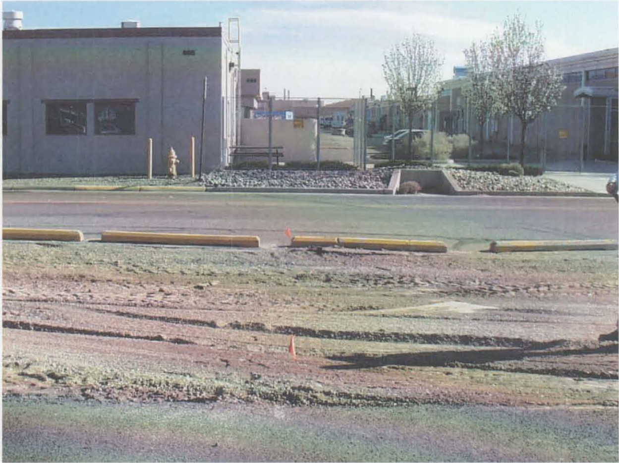
Figure 3.2-1 Two orange pinflags mark the location of the DSS Site 1101, Building 885 septic system, drain line running north from Building 885 (upper left of photo) and beneath "H" Street. View to the south. March 26, 2002
