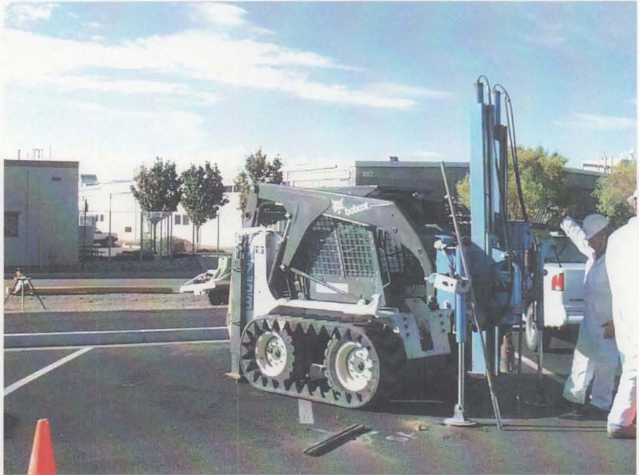
Figure 3.4-1 Auger drilling at the DSS Site 1101, Building 885 septic system seepage pit location in the parking lot north of Building 885, shown in the center-left side of the photo. View to the southwest. October 21, 2002
