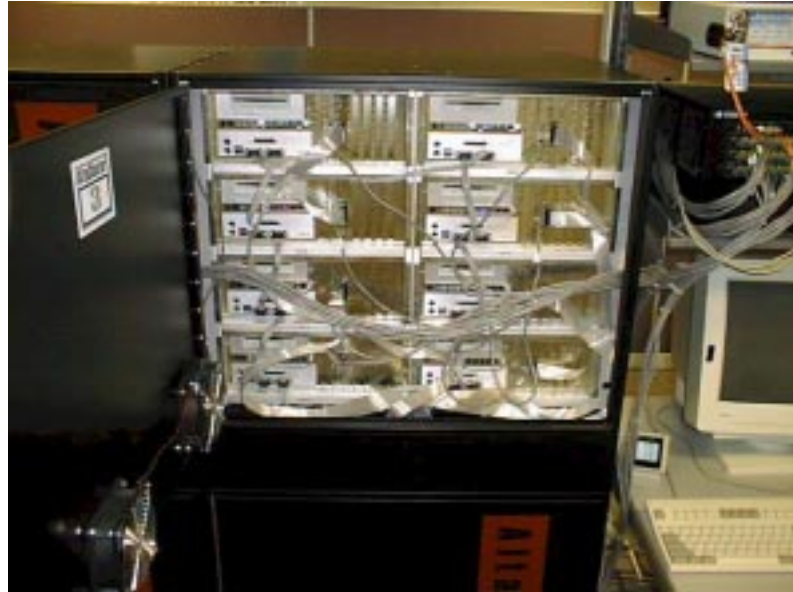
Figure 2: A Peek Inside the Roadrunner.
