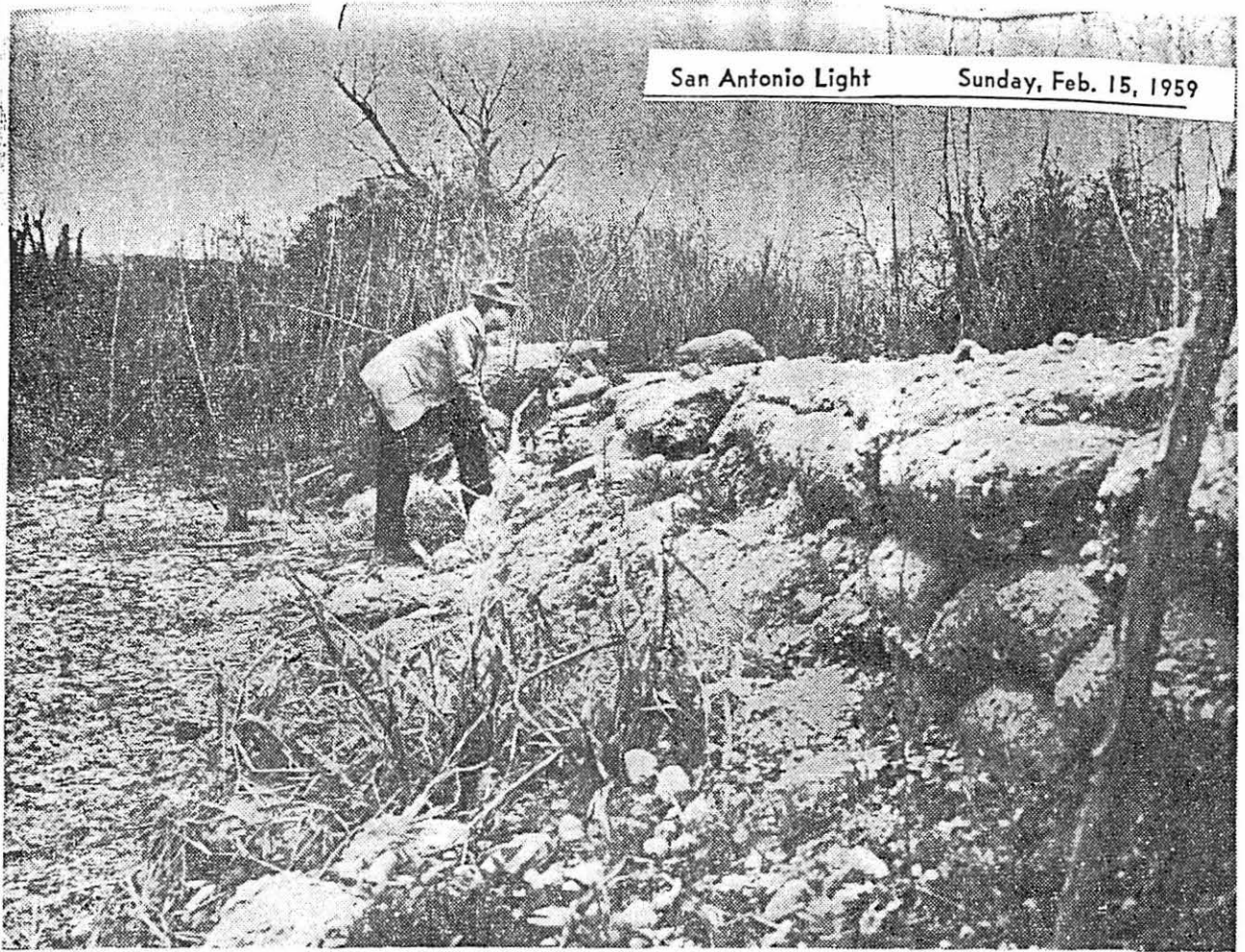
FLOOD CONTROL PROGRAM LEFT THIS OLD SPANISH DAM HIGH AND DRY Dam supplied water to the irrigating system area near Mission San Juan de Capistrano.
