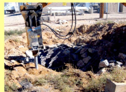
Seepage pit demolition and backfilling.
