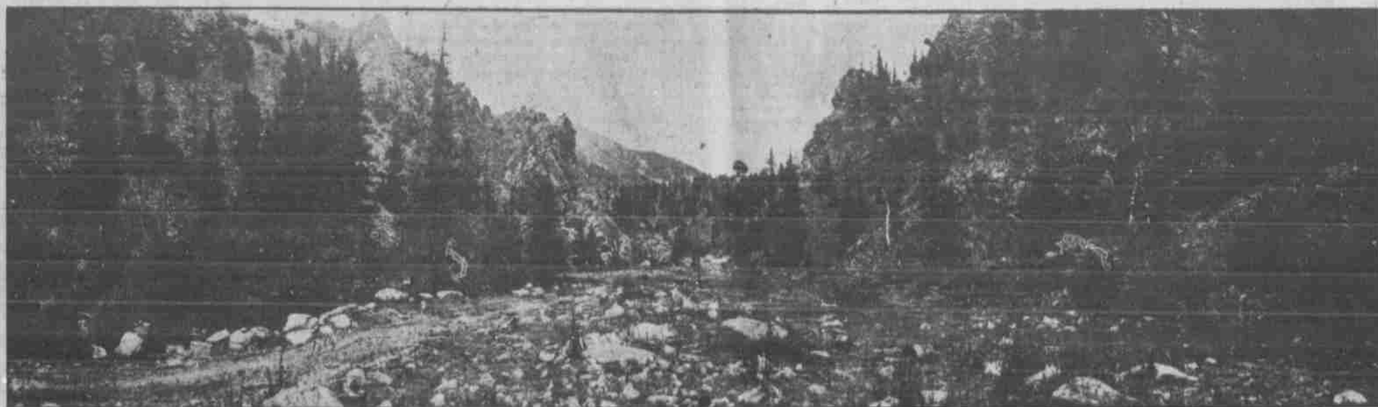
Eagle's Nest in Cimarron Canyon, where dam will be constructed that will make a reservoir holding enough water to irrigate 120,000 acres of best of agricultural land near Cimarron
