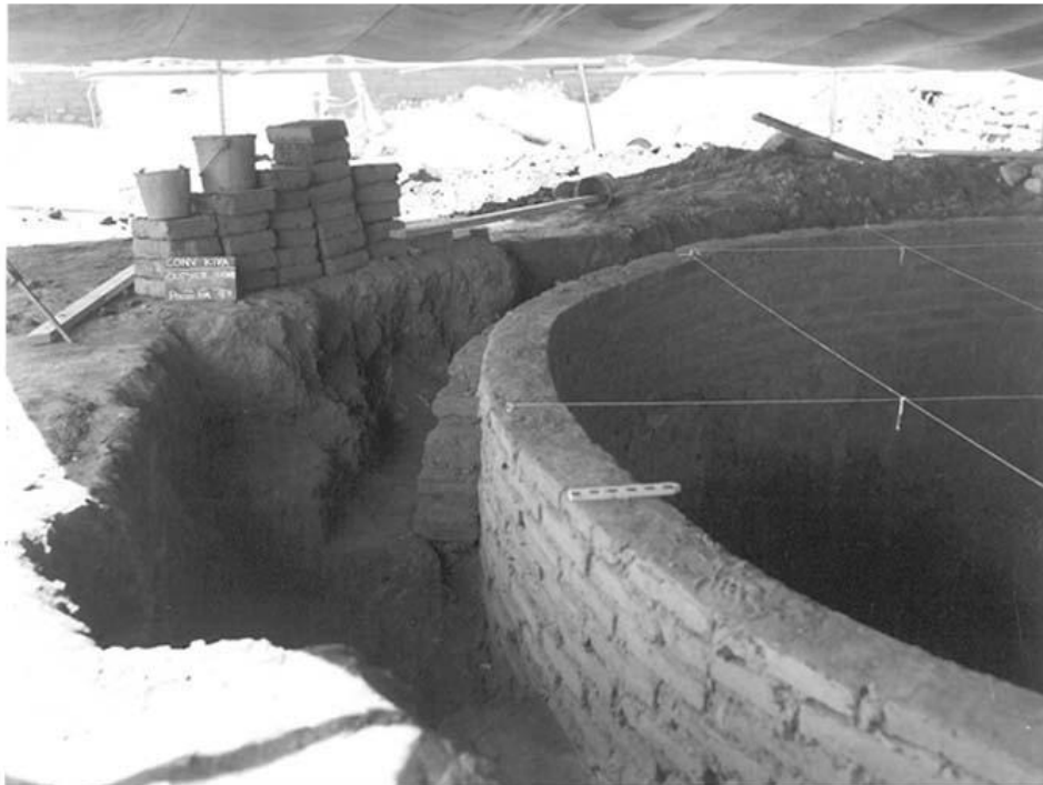
Figure 7. Photographs of stabilization and reconstruction of convento kiva in 1971 (Matlock 1971, Photos 356 and 627).
