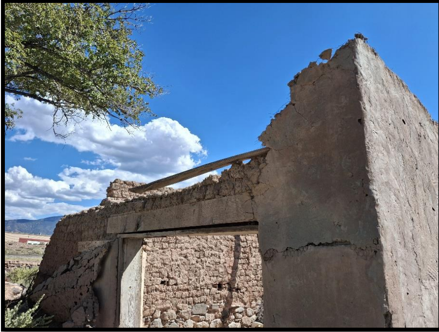
Molino at El Llanito, near Town of Bernalillo, with walls on main floor constructed of terrones
