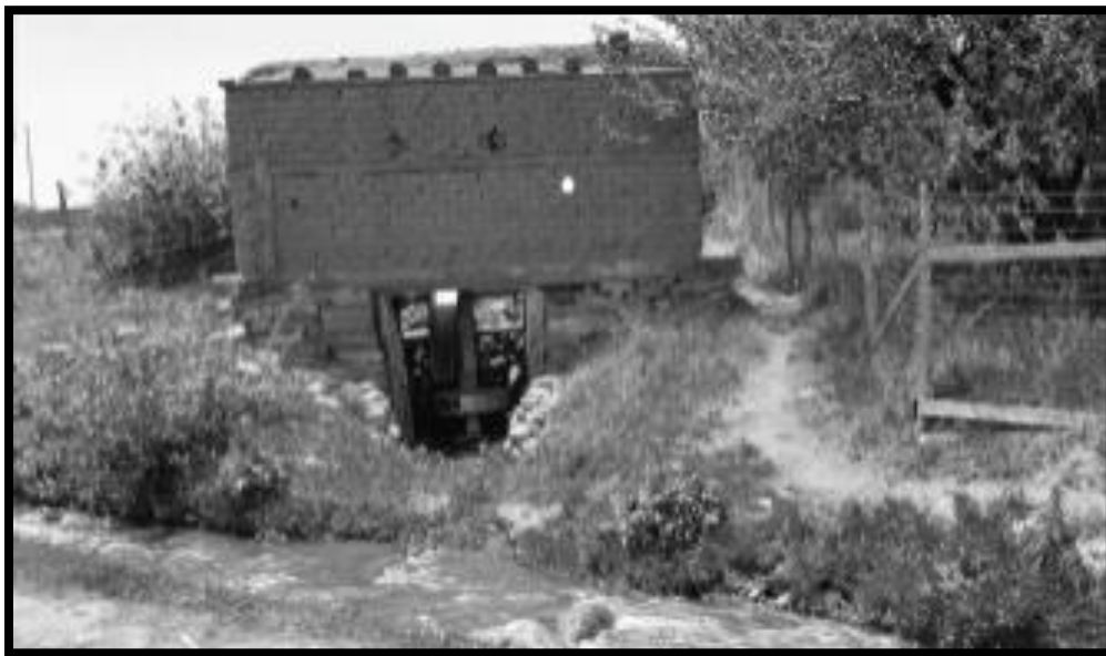
William H. Roberts, Old mill on Acequia Madre above Manhattan Street, Santa Fe, ca. 1920-1930. Courtesy of the Palace of the Governors Photo Archives, 149931 [Note the adobe construction versus the log-built design of most other mills.]
