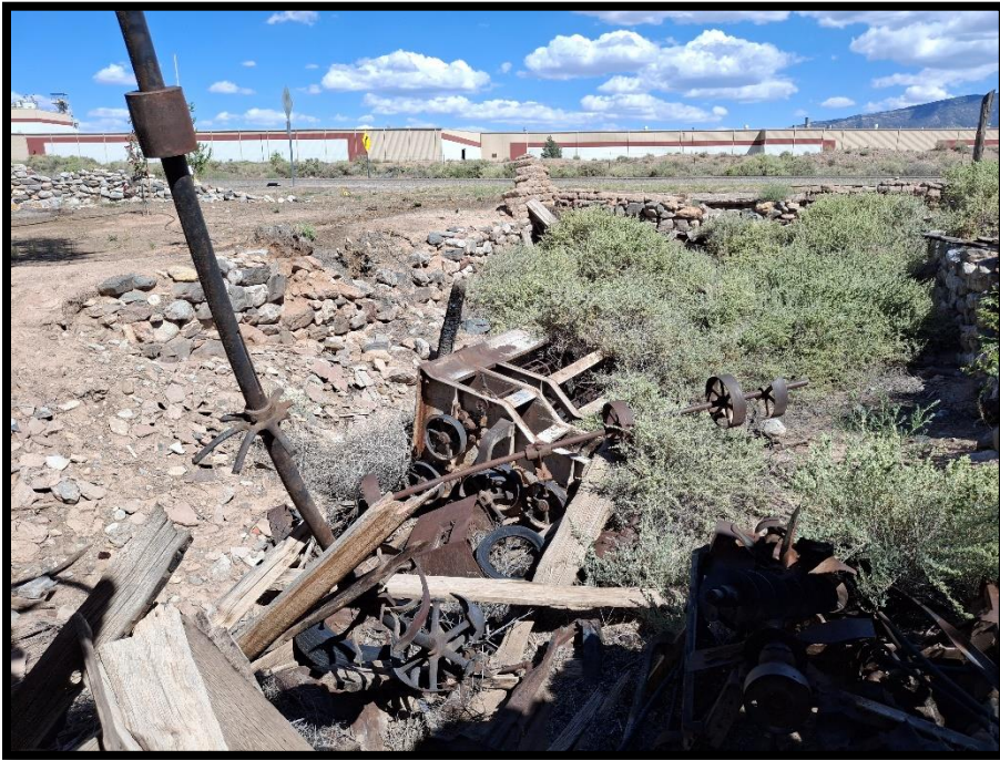
Adjacent basement floor of molino at El Llanito after collapse of walls and removal of terrones with milling equipment left behind
