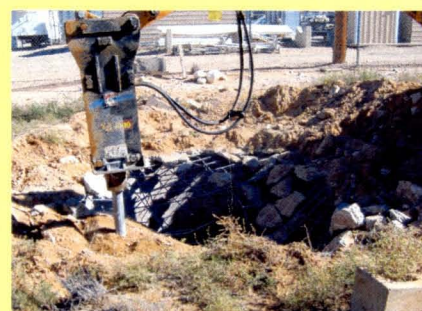
Seepage pit demolition and backfilling.
