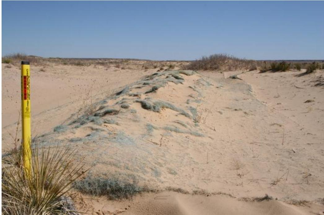
Figure 10: One year old geotextile repair, placed over sand mounded on top of exposed pipeline. Geotextile is already being torn away from repair. Photo: Knutt Peterson
