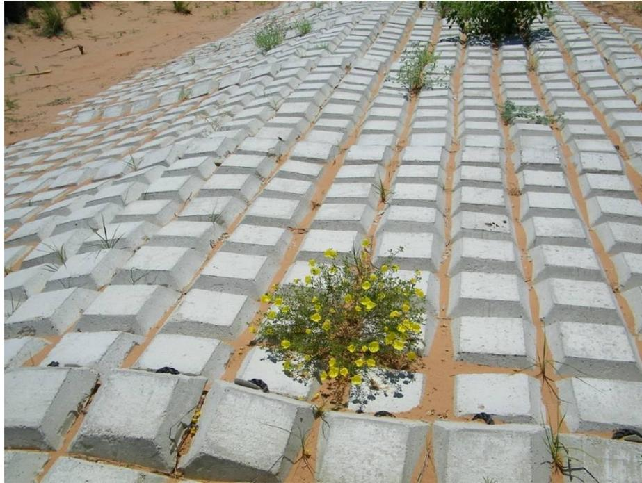
Figure 8: Articulating concrete mat at one of Submar’s testing sites in Southeast New Mexico. Photo courtesy of Submar.
