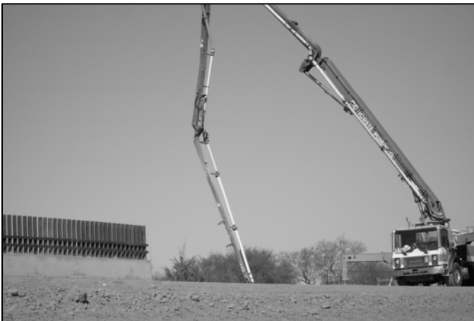
Image 6.1 Photo of the border wall under construction in Hidalgo, TX. January 2009.
