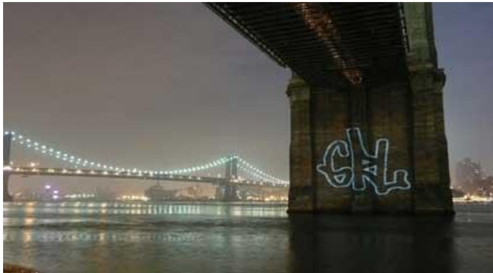
Figure 8: GRL Laser Tag on the Brooklyn Bridge, NY. 2007
