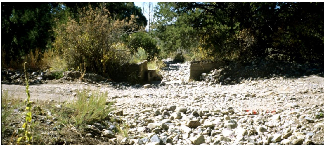
Latir Creek Compuerta (Headgate), October 1999
