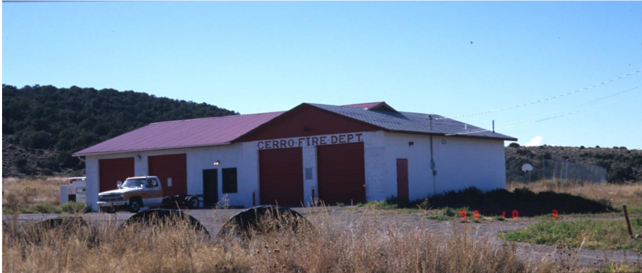
Cerro Fire Department, October 1999
