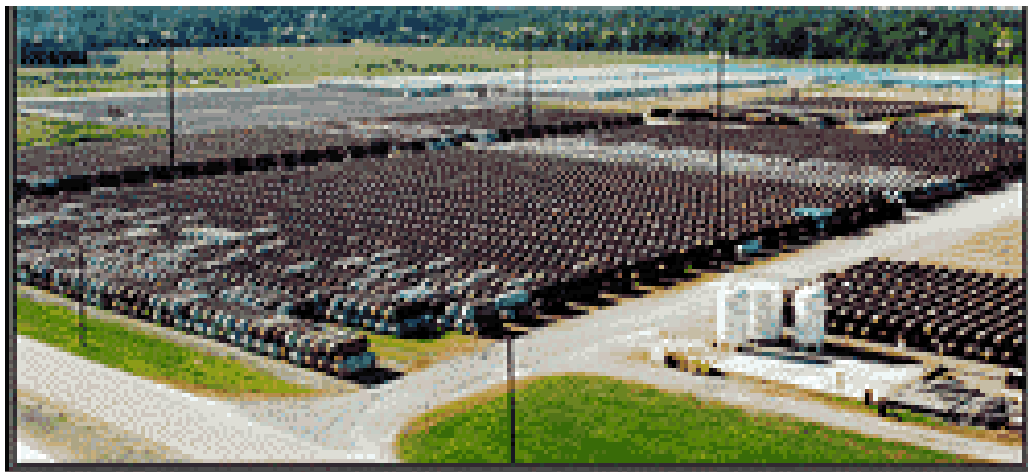
DUF 6 Cylinder Storage Yard at a Gaseous Diffusion Plant in the U.S. [ANL 2013]
