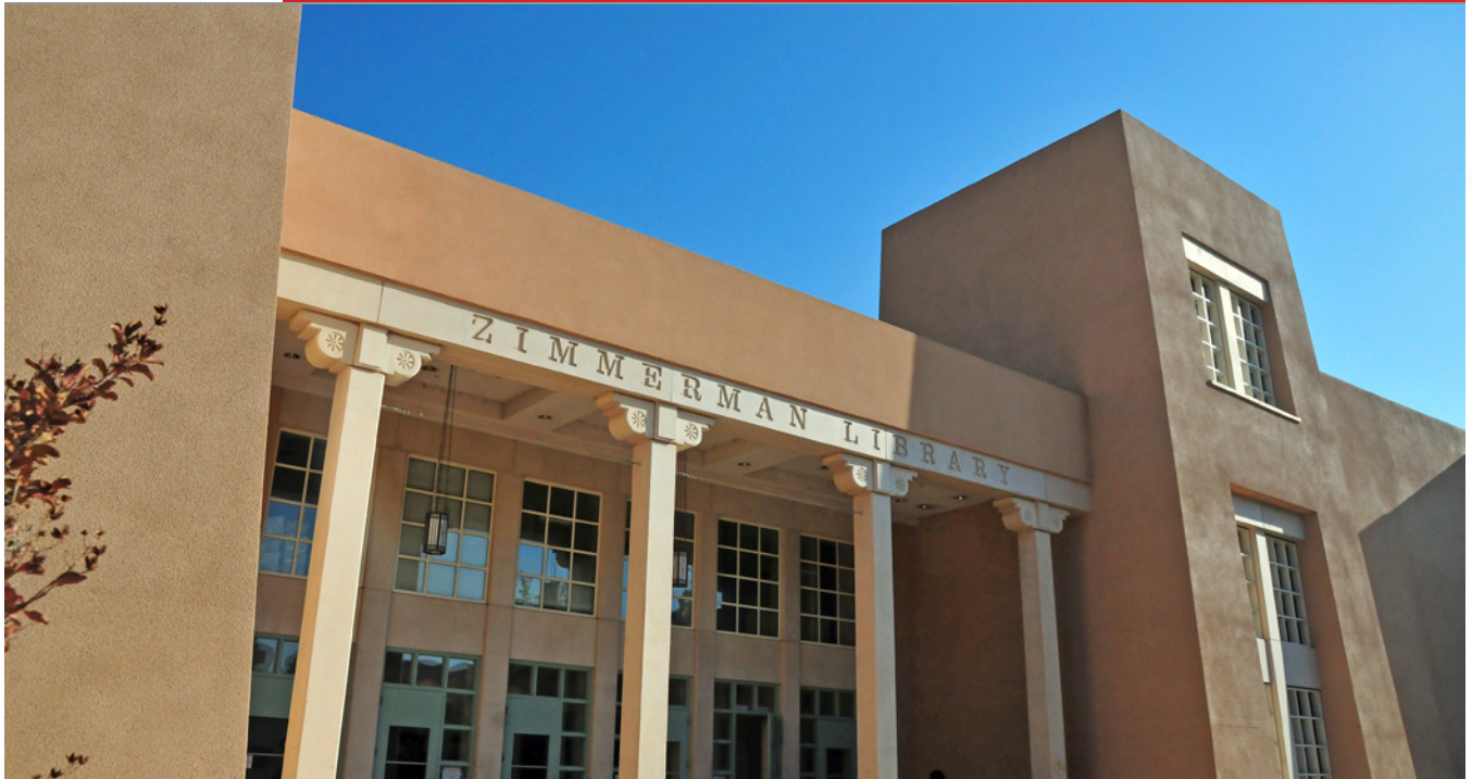
The south entrance of Zimmerman Library.
