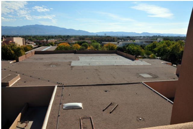
Exhibit 4. Photo of Zimmerman Roof
