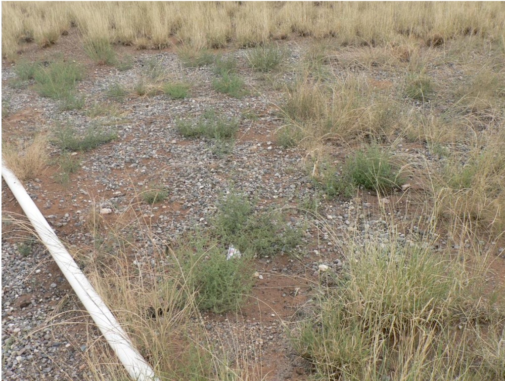
Northwest corner of cover: facing center of cover (This small area has the lowest density of native perennial plants on the cover)
