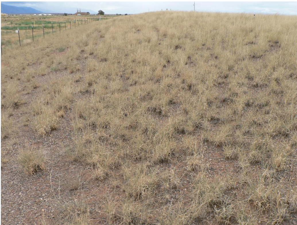
West slope of cover: northern end
