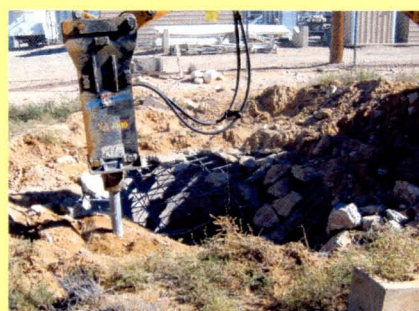
Seepage pit demolition and backfilling.
