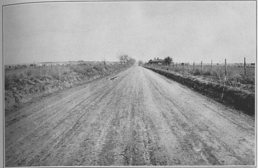
EDDY COUNTY. State Road No. 2. View taken about two miles out from Carlsbad; showing graded earth road.
