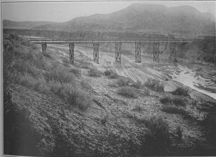
VALENCIA COUNTY. State Road No. 6. Sec. 2. Rio Puerco bridge.
