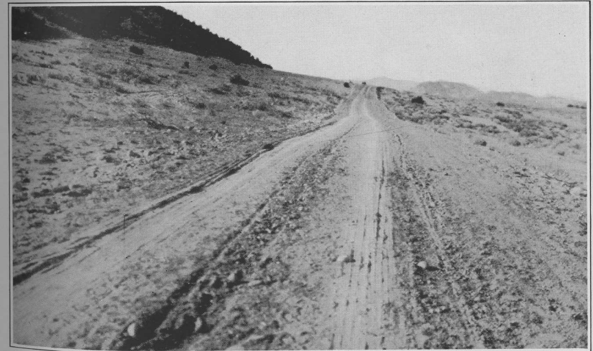
RIO ARRIBA COUNTY. State Road No. 36. Sec. 5. A graded gravel road through heavy sand on the Espanola-Abiquiu road.
