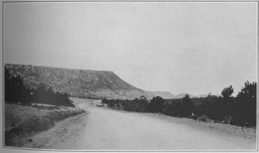
SAN MIGUEL COUNTY. State Road No. 1. Sec. 6. Limestone surfaced with motor truck.
