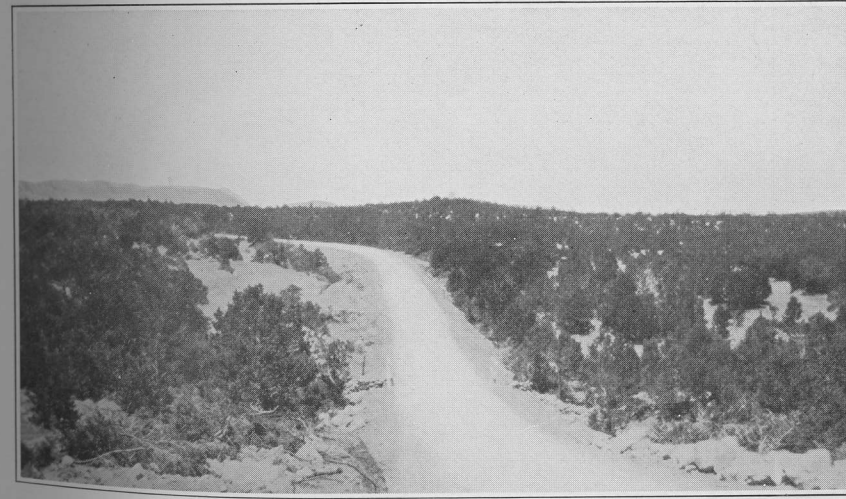
SAN MIGUEL COUNTY. State Road No. 1. Sec. 6. This road is of rock, surface of crushed limestone.
