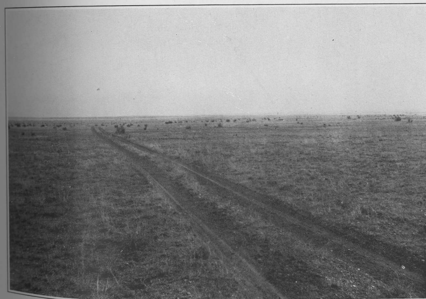
SIERRA COUNTY. Type of mesa road constructed by a drag to make the rut. This type on flat mesas can be made for about $5 per mile; does not require drainage.
