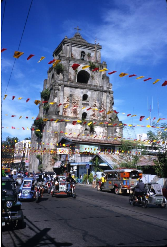
Cathedral Bell Tower at Laoag City
