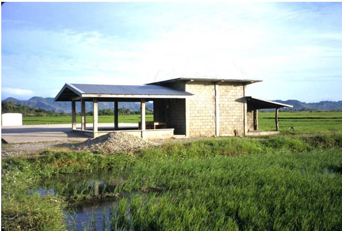
Kamarin at Zanjera Surgui: A Place to Meet and Plan Operations
