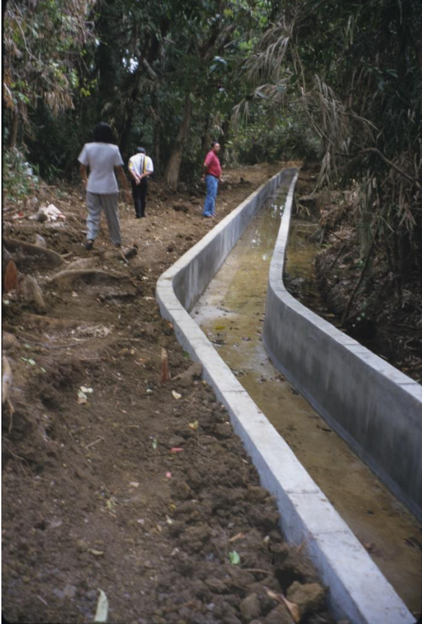
Zanjera Tadao Canal Rehab Project at Springs
