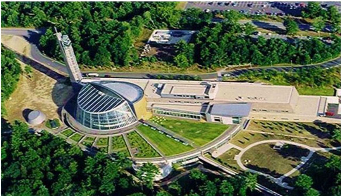
Aerial View of MPMRC (Photo by American Hydrotech Inc. 2009)
