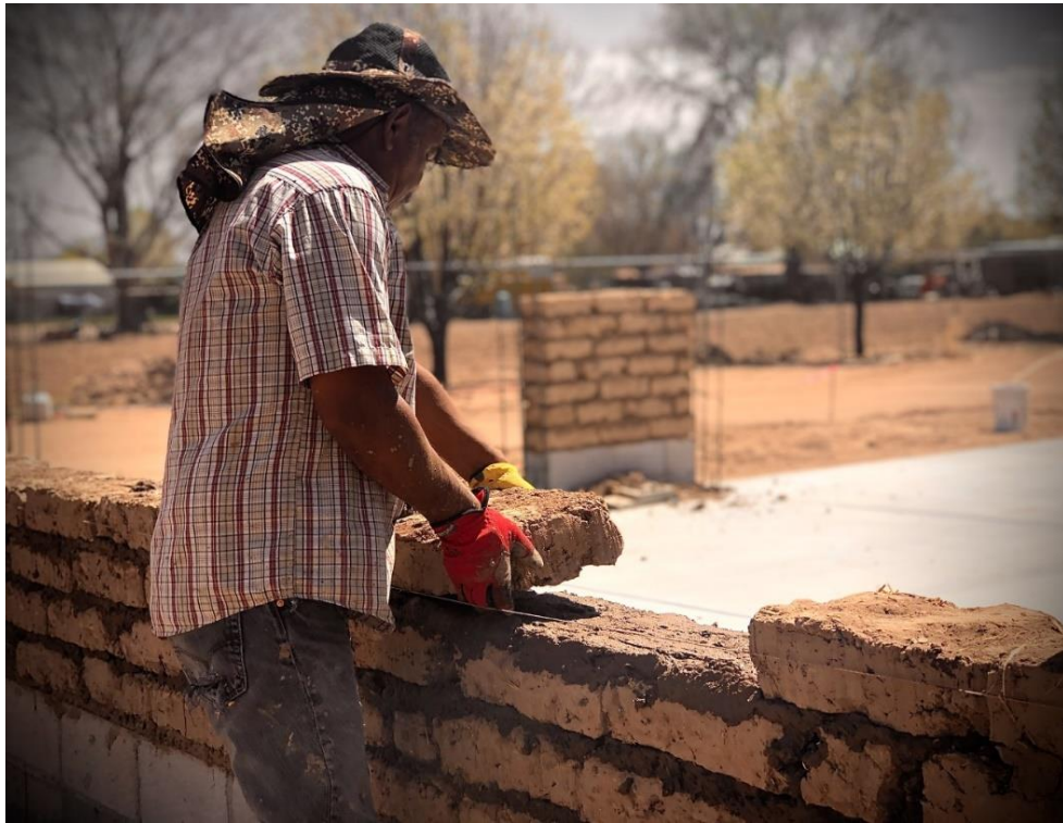
Adobero forming exterior walls
