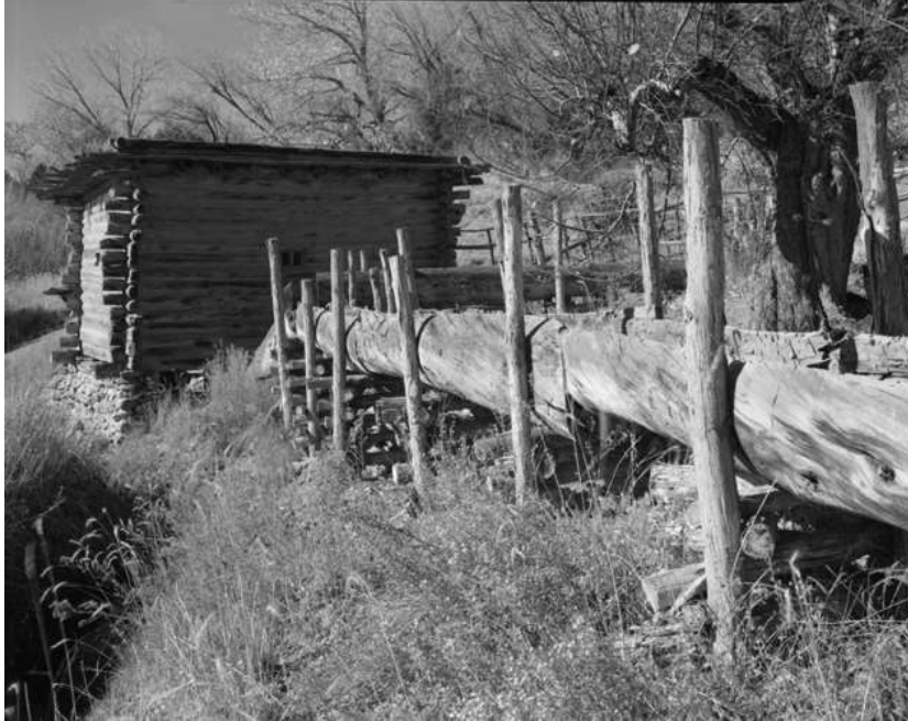
Title: LA CANOA ELEVADA: Trough of hollowed log, elevated on log structure. - La Cienega Acequia, Truchas Molino at Rancho de las Golondrinas, Santa Fe County. Creator(s): Stupich, Martin , creator. Date Created/Published: 2007
