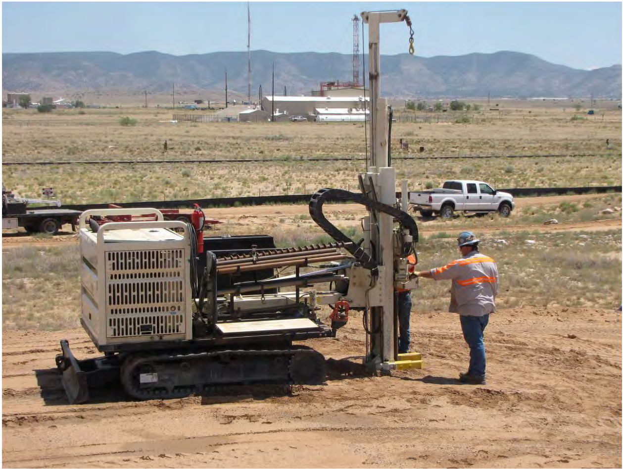
Figure 2-1 Pushing the Geoprobe rods to the target soil-vapor sampling depth at the soil-vapor well MWL-SV02 location, August 5, 2009 (view to the southeast).
