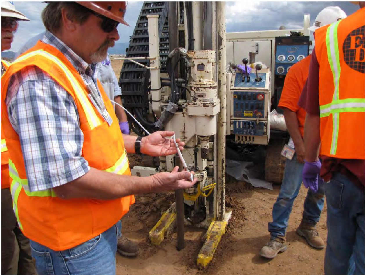
Figure 2-2 Geoprobe soil-vapor implant attached to 1/4-inch-diameter polyethylene tubing, which was inserted into the Geoprobe rods and lowered to the required soil-vapor sampling depth at soil-vapor well MWL-SV02 location, August 6, 2009 (view to the south).
