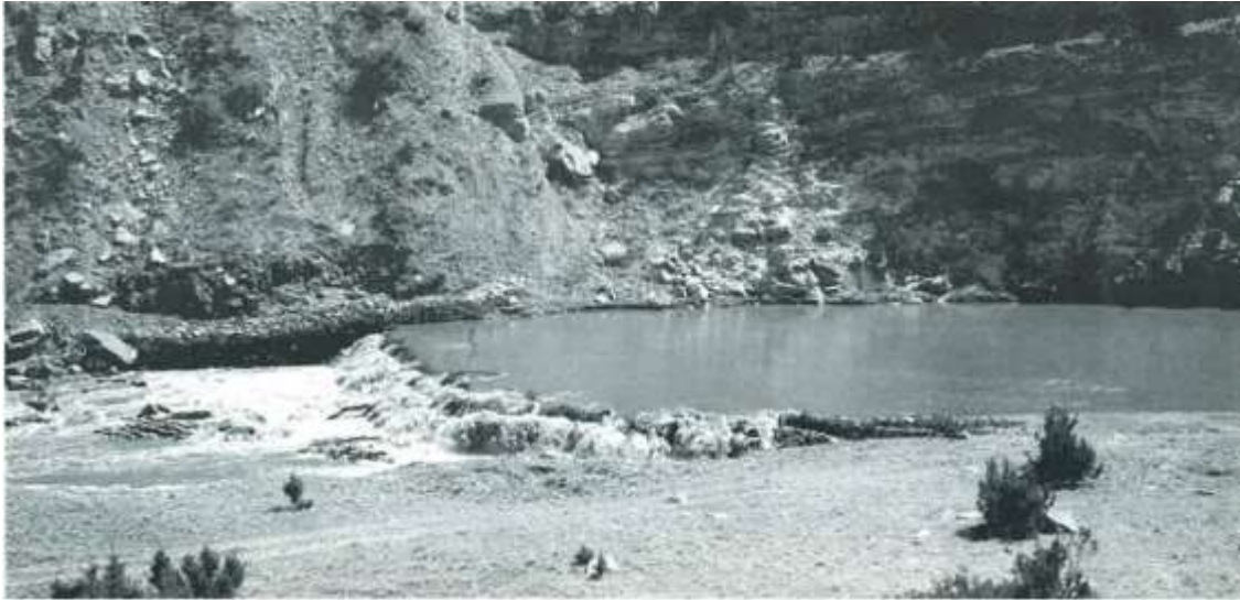
El Cerrito NM 1941 Old Dam of Brush and Rocks. Irving Rusinow Photo in NARA
