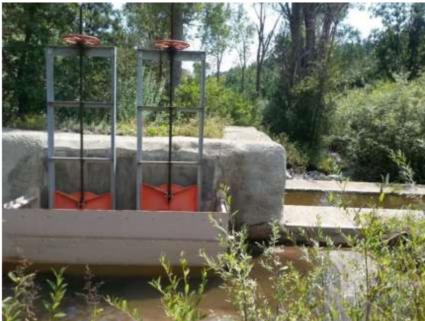
Encinal & Cañoncito Community Ditches Trans-Basin Diversion Gates Dividing Water for Use in Each Community. September 2017
