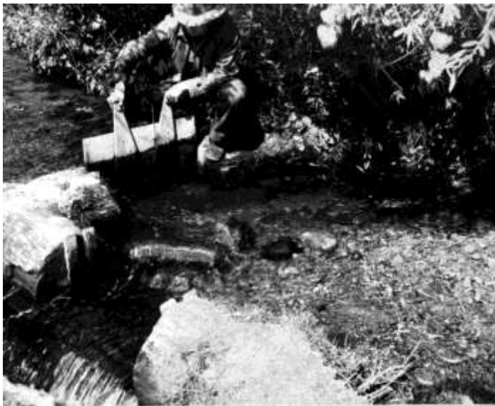
Wood Compuerta Río Arriba County 1938. Museum of NM Photo
