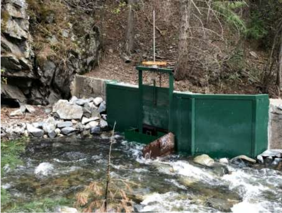
Río Hondo La Cuchilla Diversion at Valdez NM. New Headgate. Sylvia Rodríguez Photo May 2021
