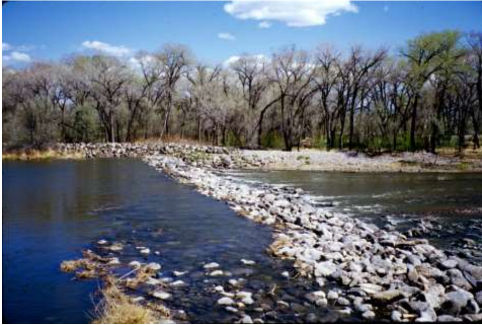
Río Grande Rocks Topping Concrete Base for Acequia at El Guique NM. April 2000
