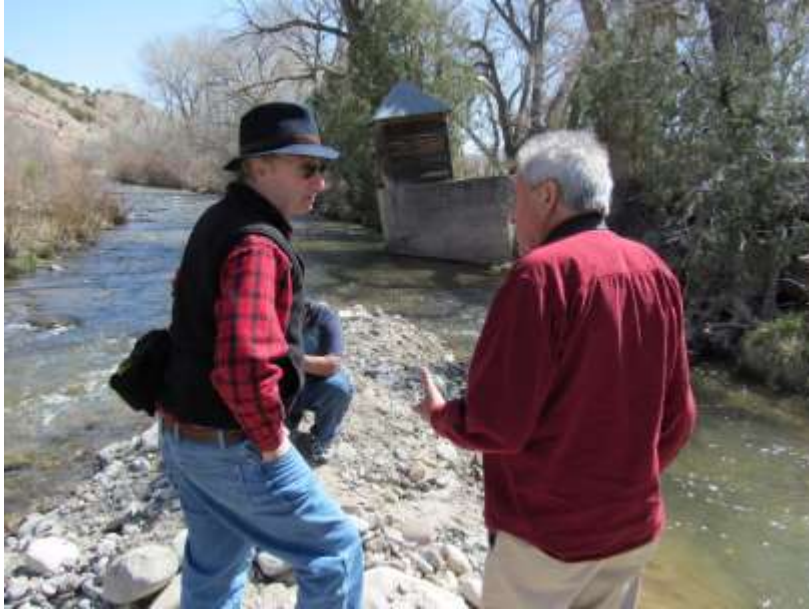
Río Embudo Rock Diversion at Low Flow. Tom Glick and Estevan Arellano April 2011
