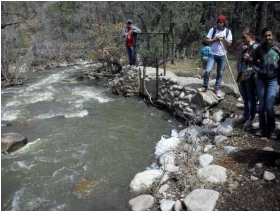
El Rito NM Presa of Stone Alignment & Chain Hoist Gate during High Flow. March 2012
