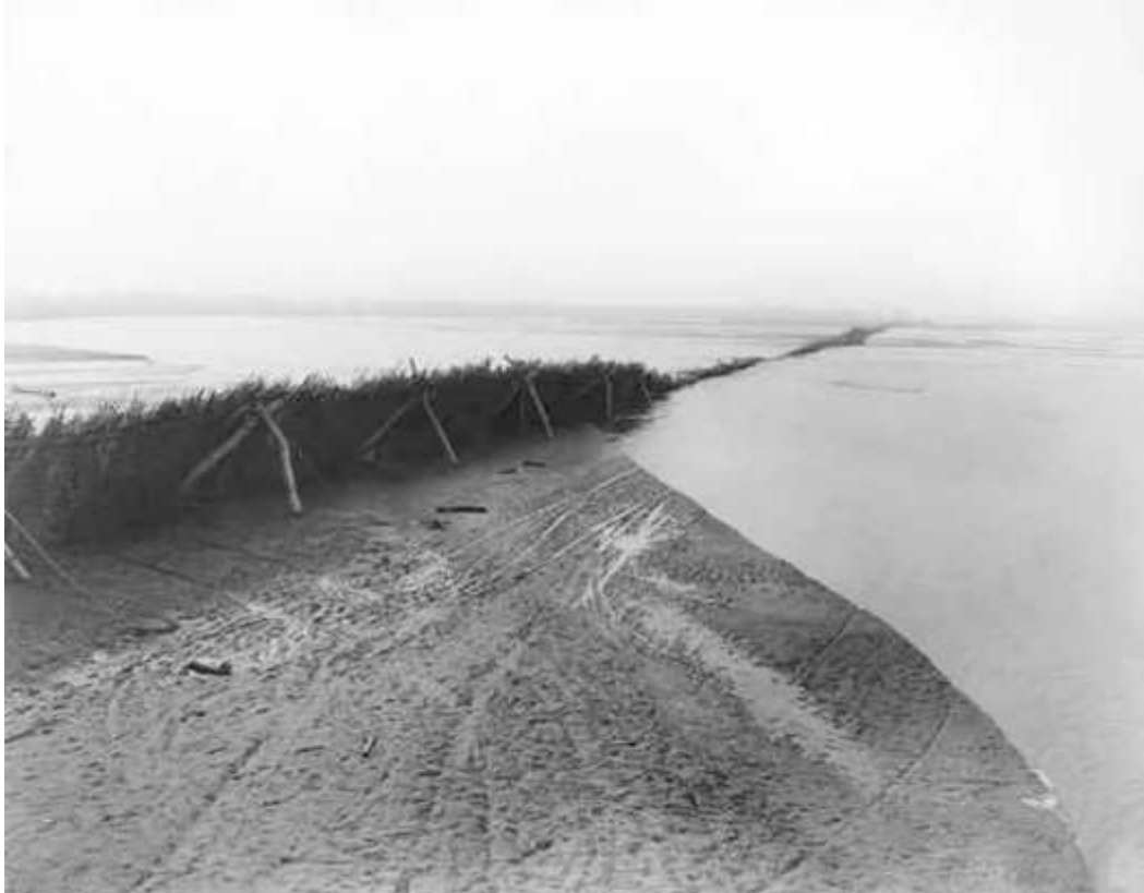
Wing dam at sandbar. View of Río Grande from Isleta Highway Bridge 1931. Courtesy of the Middle Río Grande Conservancy District, New Mexico. Note the use of posts, willows and mesh to support the structure.
