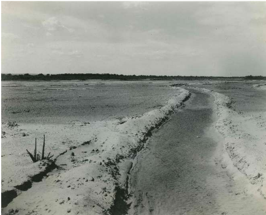
Acequia heading extended into river channel at Isleta Pueblo July 1930. Courtesy of the Middle Rio Grande Conservancy District, New Mexico.
