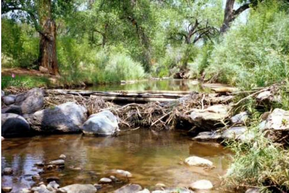
Río Jémez Presa Logs and Boulders for Jémez Springs South Side Upper Ditch. August 2000
