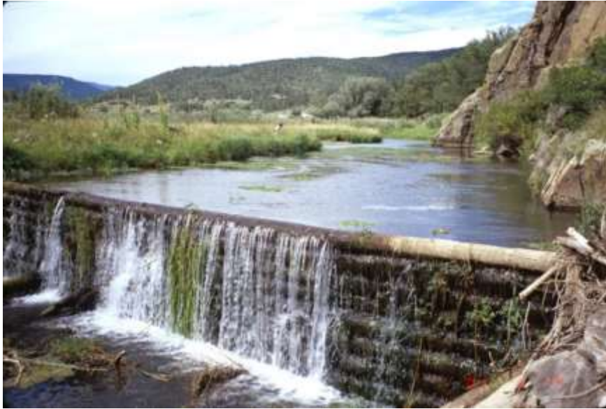
Río Mora Presa of Logs Diverting Water for Hydro-Power Roller Mill at Cleveland NM. September 2000
