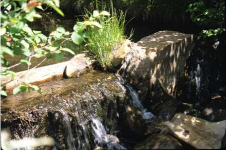
LeDoux Small Dam Dividing Water San José and La Isla Acequias. Poured Concrete Base & Logs. June 2000
