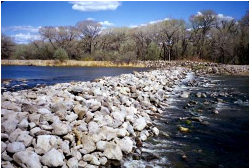
Río Grande Rocks Topping Concrete Base for Acequia at El Guique NM. April 2000
