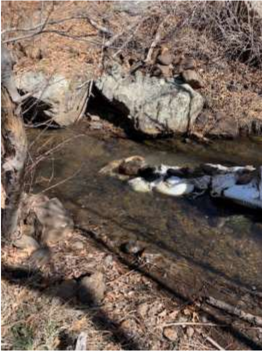
LeDoux Oldest Diversion of Rocks and Bags Filled with Dirt for Three Acequias. Harold Trujillo Photo April 2021
