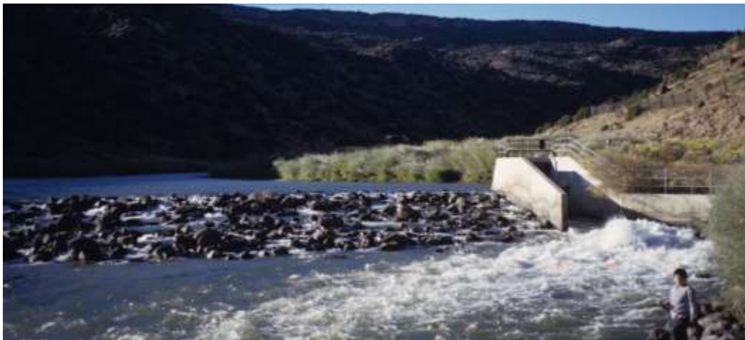
Velarde Modernized Dam and Floodgate on the Río Grande. October 1999
