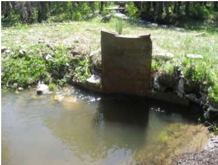
Trans-Basin Acequia de la Sierra Headgate for Holman in Mora Valley NM. June 2008
