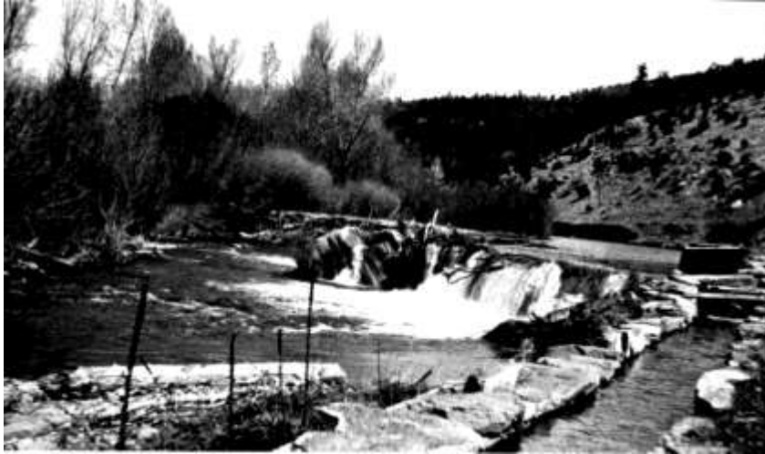
Brush and Rock Dam on the Río Pecos NM c. 1917. Museum of NM Photo
