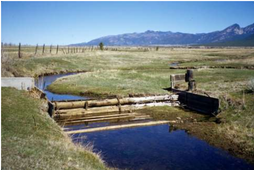
El Prado Presa of Logs for Acequia del Medio Near Buffalo Pastures Taos NM. April 2000
