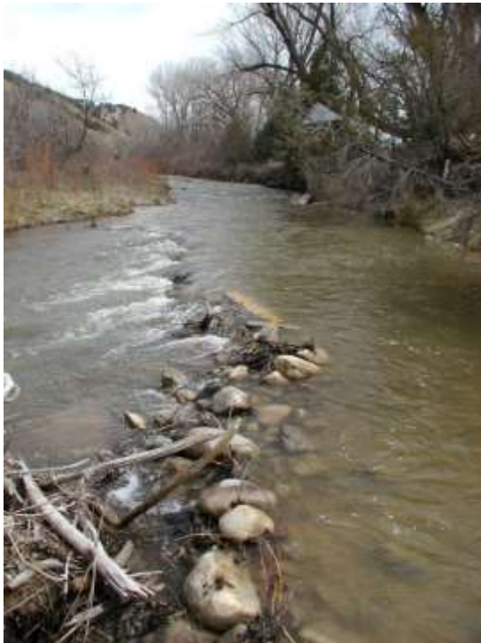
Río Embudo Rock Diversion during High Flow. Denise Bleakley Photo March 2005
