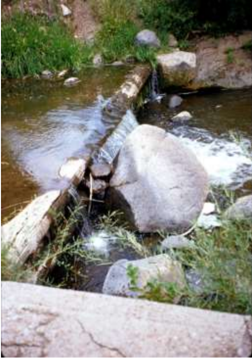
Río Jémez Log and Boulder Presa for West Side Ditch at Jémez Springs NM. August 2000
