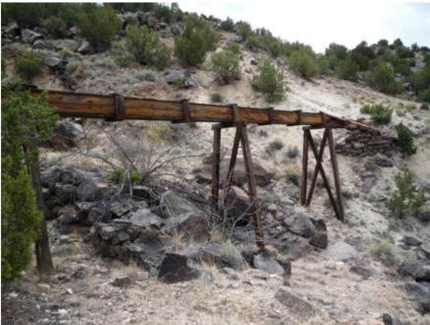
Trestle support for community acequia pipeline in a wooden box at La Bajada NM. Arnold Valdez Photo 2009
