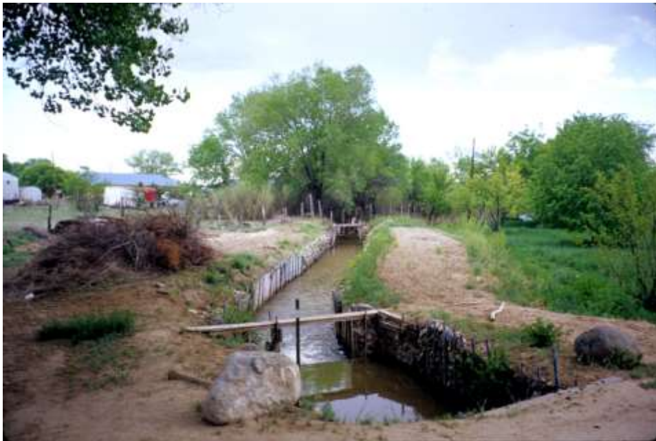
Río Chama Reinforced Ditch and Footbridge at Chamita. May 2001
