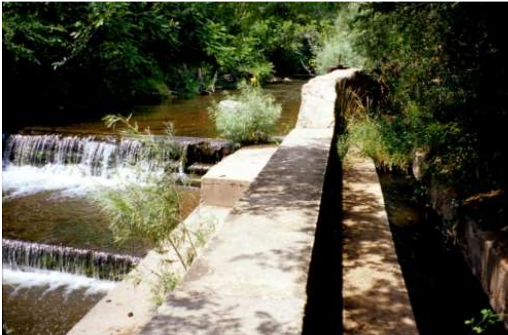
Río Jémez Log Presa for Jémez Springs Community Ditch. August 2000
