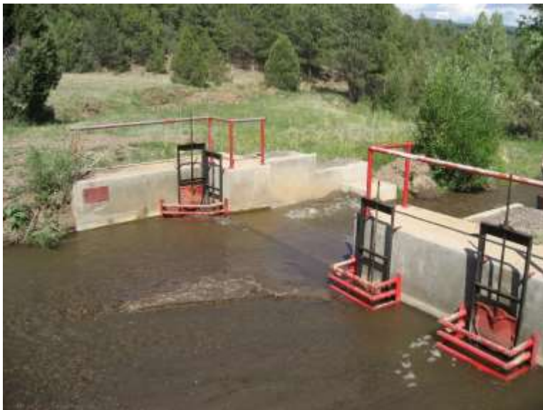
Trans-Basin Acequia de la Sierra Gates at Holman NM. June 2008
