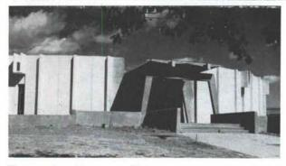
The new Los Alamos, N. M. High School Learning Center featuring 8' single tee wall panels, precast canels  $\mathcal{G}$  prestressed entry roof tees, all exposed precast concrete received an applied ARCHITECTURAL COATING.
