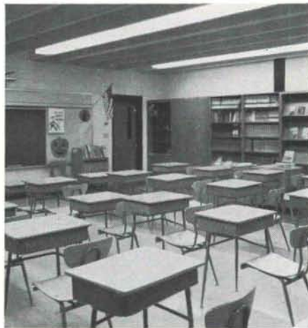
Classroom with ceiling of exposed double-tees and concrete masonry walls
