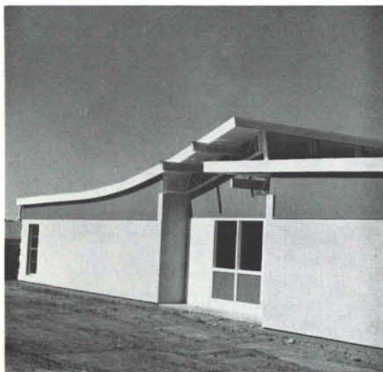
Penasco Elementary School — Penasco, N. M. Harold R. Benson, A.I.A. Architect
