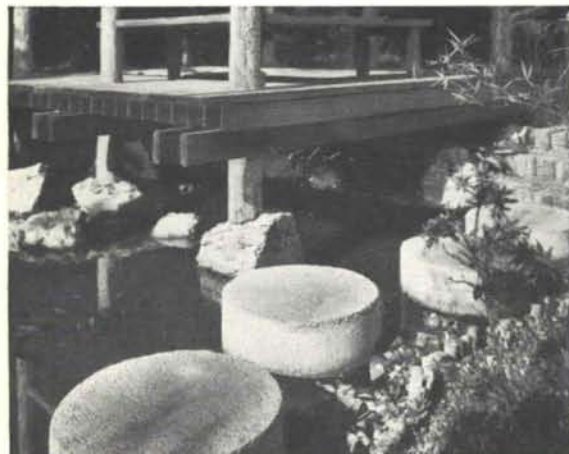
Rugged concrete "islands" provide attractive access to tea house. Landscape Architect: Phil Shipley.
