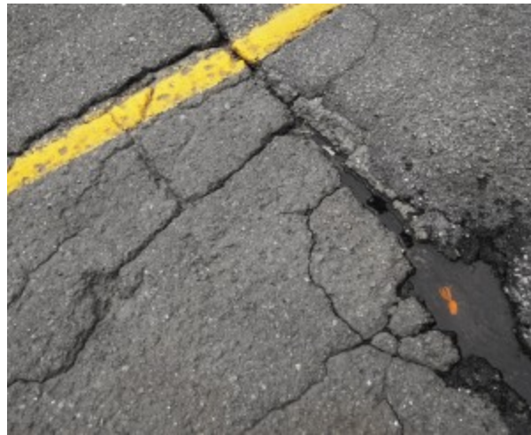
Figure 2.3 Moisture damage in asphalt concrete
