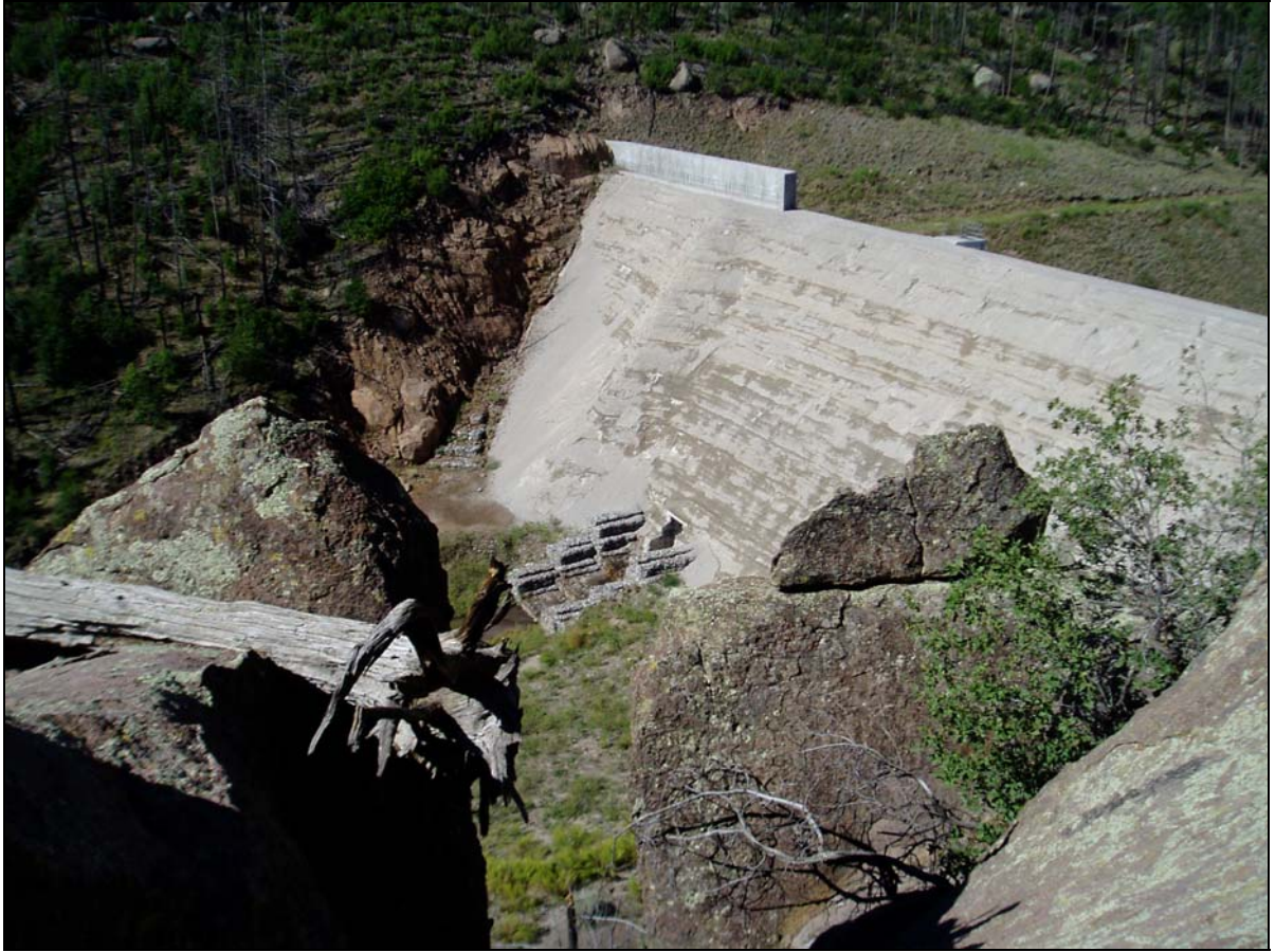
Figure 6. View of PFRS outlet
