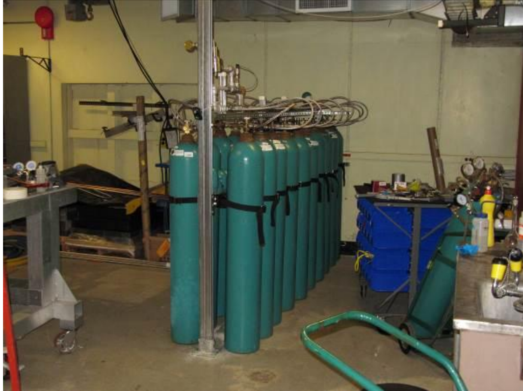
Figure 1.2: Photograph of the Helium Gas Bottle and Gas Manifold Used During the Once-through Helium Gas Cooled Thermal Test Using the Electron Accelerator at ANL in March 2011
