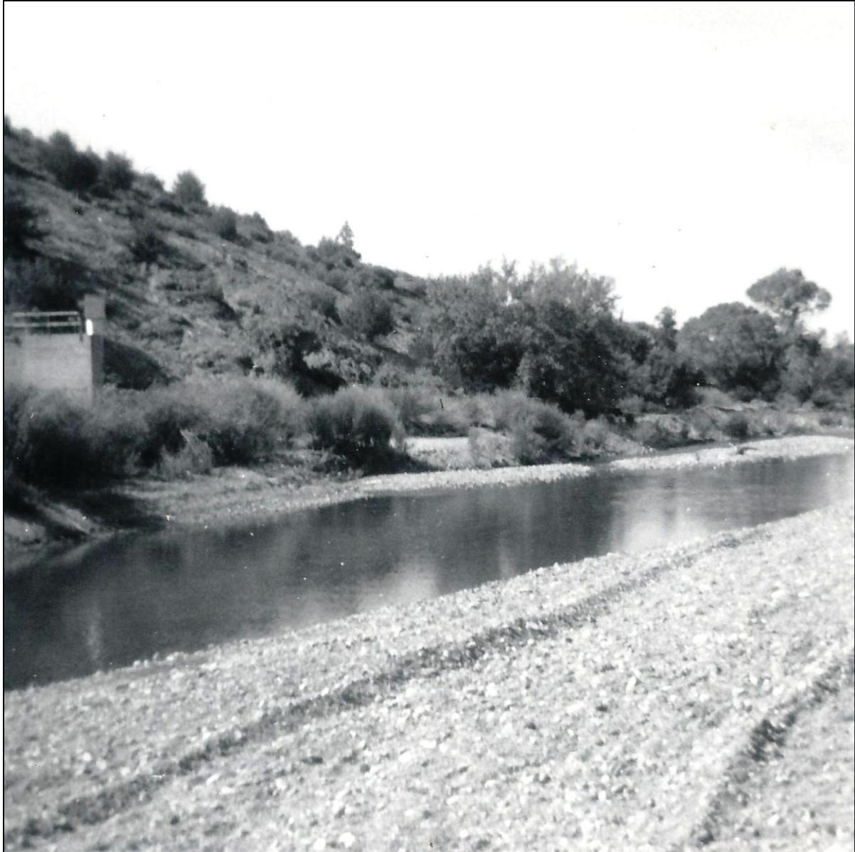
Figure 5. 1972 photo at the upstream end of the study site, looking downstream from the right bank with the stream gage structure visible on the left. Note that unsorted gravel in the foreground has distinct ridges, and appears to be fill material recently-graded with heavy equipment. This is presumably the result of channelization work of 12/17/1971 referred to in Table I. Flow direction is from left to right. From USGS photo archive, New Mexico Water Science Center, Albuquerque, NM.
