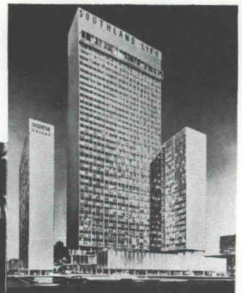
SOUTHLAND CENTER, DALLAS, TEXAS Welton Becket, F.A.I.A. and Associates. Architects & Engineers. J. W. Bateson Co., Inc., General Contractor. Atlanta Tile & Marble Co., Tile Contractor
