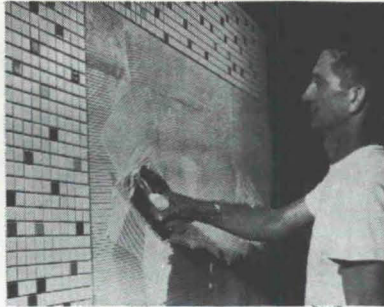
No special preparation of back-up needed. Here TILE-SET is floated on dry portland cement brown coat. Special notched trowel gives proper thin-bed mortar thickness.
